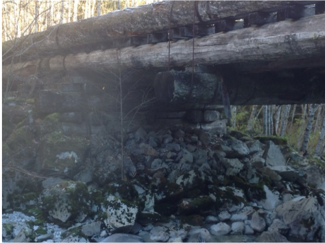
right pier crib
