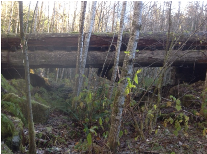
upstream profile of 2nd span
