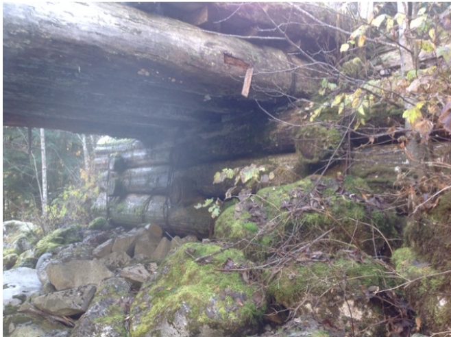
Right Bank Abutment when facing downstream
