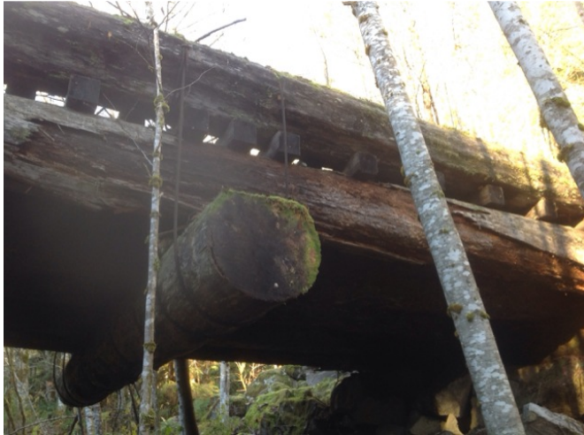
typical stringer condition
