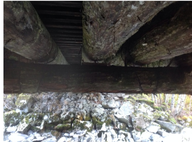
first span loose needle beam
