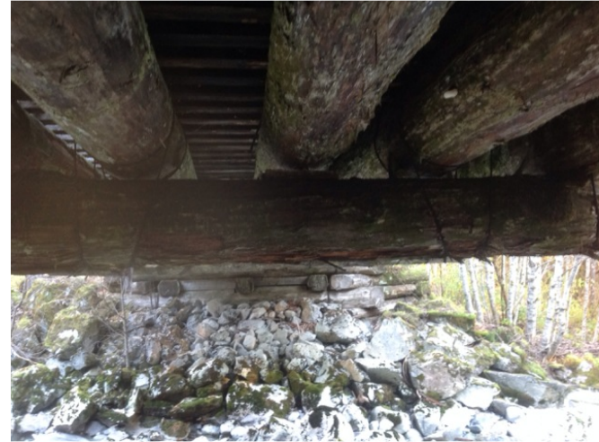
first span stringers
