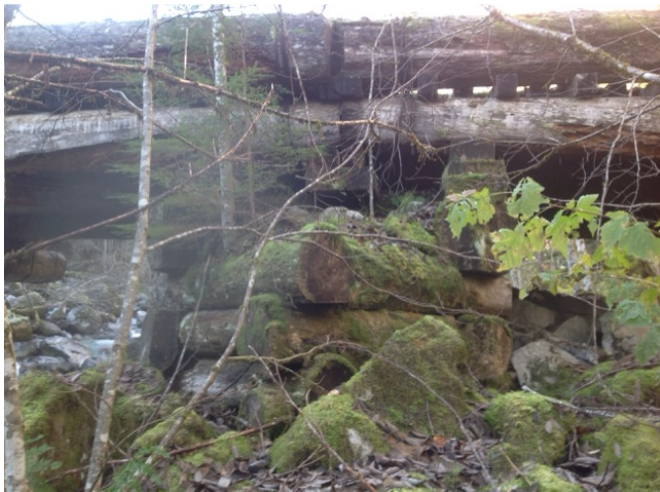
downstream profile of pier
