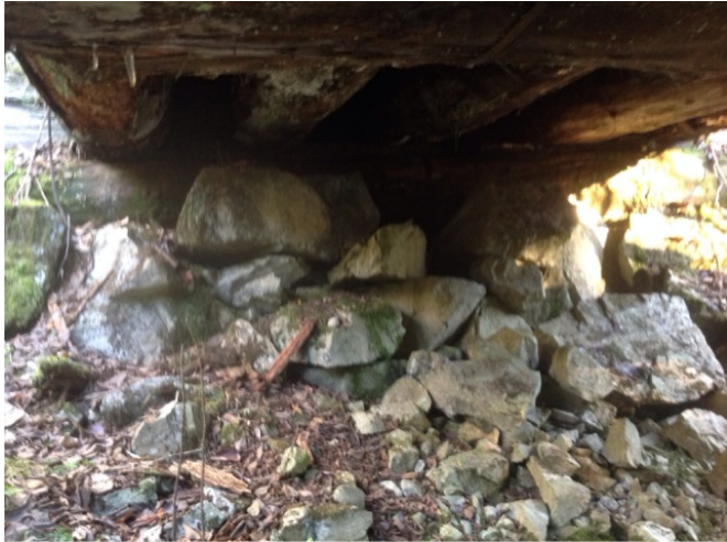
Left Bank Abutment when facing downstream
